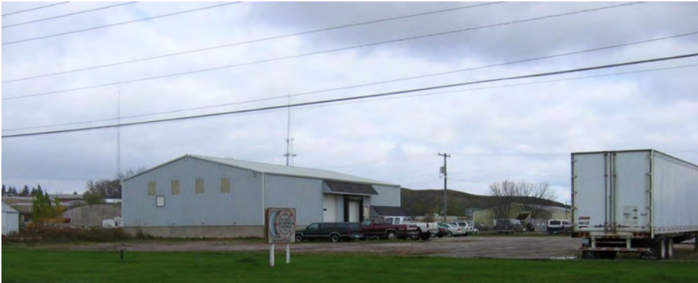
Before - Underutilized Industrial Park
