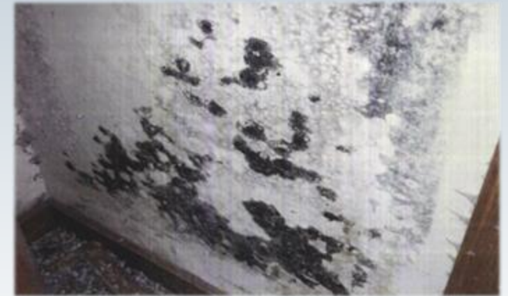
Mold growth on water-damaged wall
