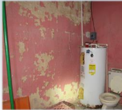
Deteriorating lead-based paint
