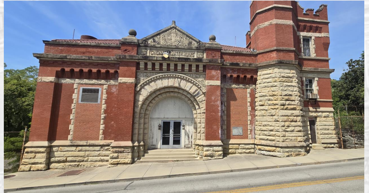
Eden Park Pump House TBA in Cincinnati, Ohio
